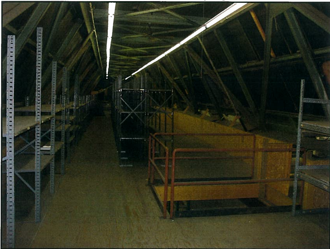
VIEW OF MEZZANINE SPACE
